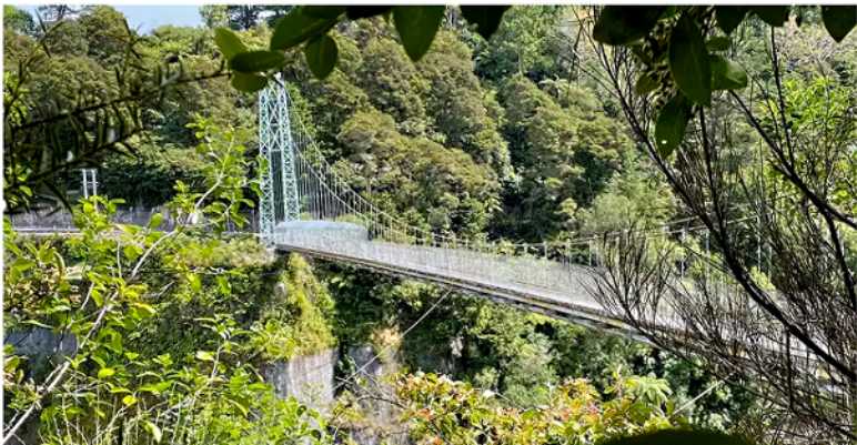
THE ARAPUNI SUSPENSION BRIDGE ABOVE THE ARAPUNI POWER STATION AND DAM
